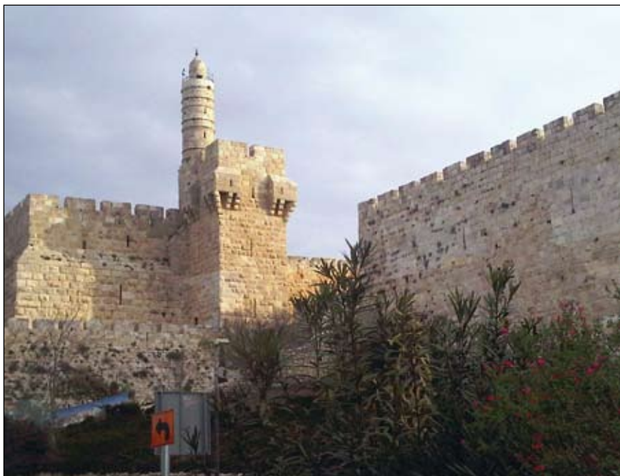
The walls surrounding Old Jerusalem show signs of the centuries of rebuilding. This is the tower at Jaffa Gate.
